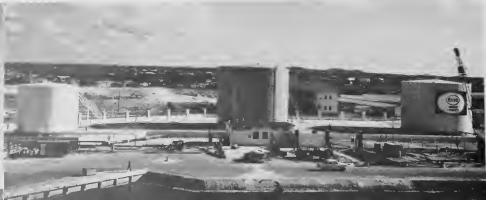
THE TERMINAL building is flanked by three storage tanks which have a total capacity of about 50,000 barrels. Three grades of bunker fuels are available to ships calling at Oranjestad Harbor.
